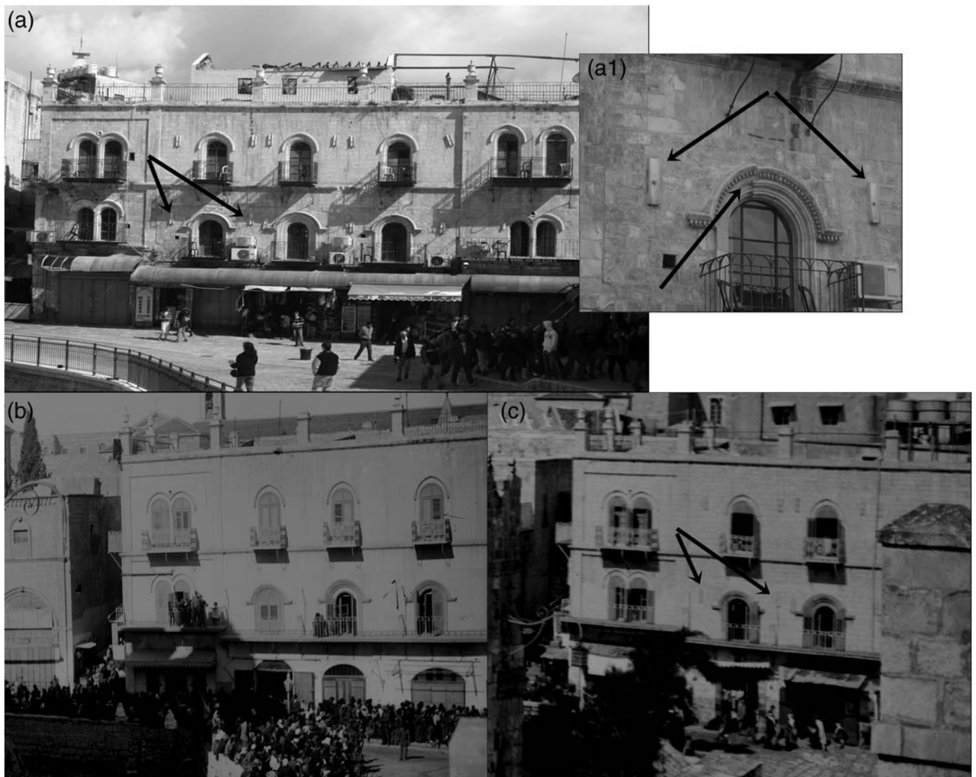
▲ Figure 4. Petra (Amdursky) Hotel: (a) present-day façade: 12 white massive iron rails identified on the second and third floors. A noticeable crack is seen above the window on the second floor (see arrows in magnified image). (b) December 1917, during the proclamation of General Allenby (reprinted from American Colony Photograph Department, Allenby's proclamation being read, Jerusalem; G. Eric and Edith Matson Photograph Collection, Library of Congress, Prints & Photographs Division, 1917, LC-DIG-matpc-08011). The front wall of the hotel does not exhibit any apparatus or cracks. (c) After 1934 (reprinted from American Colony Photograph Department, The Towers of David & Hippicus , Jerusalem; G. Eric and Edith Matson Photograph Collection, Library of Congress, Prints & Photographs Division, 1934-1939b LC-DIG-matpc-00448). The iron rails are clearly observed.
