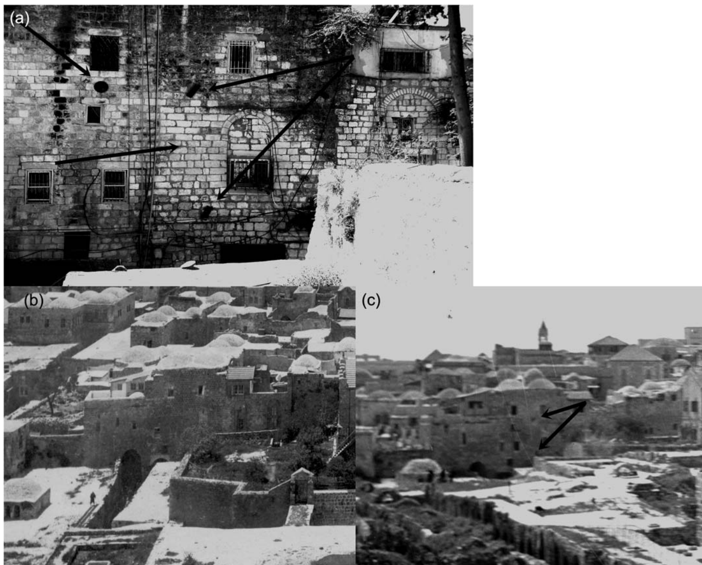
▲ Figure 5. The corner of Saint James and HaYehudim Streets: (a) current status (April 2011): both short rails and round clamps (see arrows) over the wall are visible. In addition, cracks are apparent in the same wall (marked by an arrow). (b) From the Church of the Redeemer, 1898, neither anchors nor cracks are visible (reprinted with permission from B. Hentschel, Panoramic view, Church of the Redeemer, Jerusalem, Leipzig: Yeri Rimon Collection, 1898 B. VIII). (c) Dated between 1934 and 1939 (reprinted from American Colony Photograph Department, Old City, Jerusalem, Jerusalem: G. Eric and Edith Matson photograph collection, Library of Congress, Prints & Photographs Division, 1934–1939 LC-DIG-MATPC-17817). Note that the round clamps do not appear.
