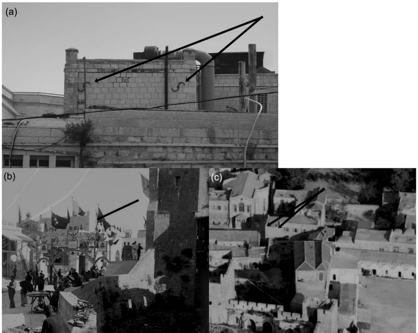
▲ Figure 8. S-shaped anchors on the Alexander building, Christ Church: (a) April 2011, facing west toward the David Tower. (b) Jaffa Gate area (reprinted from American Colony Photograph Department, moat around the Tower of David, Jerusalem; G. Eric and Edith Matson Photograph Collection, Library of Congress, Prints & Photographs Division, 1898–1946 LC-DIG-matpc-08547). The date of the photograph is vague. The wooden cabinet at the entrance to the David Tower that was removed before 1925 implies, however, that the photograph was taken prior to the earthquake. (c) Air photo of the area from 1931 (reprinted from American Colony Photograph Department, Air views of Palestine. Jerusalem from the air (Old City). Jaffa Gate and Citadel, looking east along David Street, Jerusalem; G. Eric and Edith Matson Photograph Collection, Library of Congress, Prints & Photographs Division, 1931 LC-DIG-matpc-22146). The two S-shaped anchors are marked by arrows.
