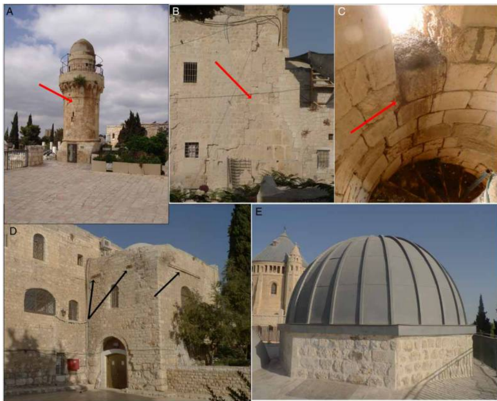
Fig. 4. Views of King David's sepulchre and visible damage (noted by red arrows): (A) the shaft of the minaret; (B) Damaged wall beside the eastern entrance facing the Muslim cemetery; (C) inner spiral stairs of the minaret. Note the damage to the inner stones; (D) Supporting iron anchors on the southeast corner of the complex (black arrows); (E) Ribbed dome on the roof above the Coenaculum (photographs: M.Z.).
