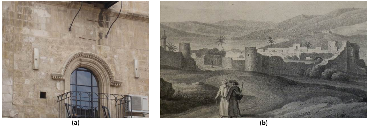
Figure 1. Data used for resolving damage: (a) Iron anchor on collapsing walls in Jerusalem after the 1927 earthquake (photograph: M.Z); (b) an old drawing of Bernatz (1839) portraying the damage to Tiberias walls after the 1837 earthquake [14]
